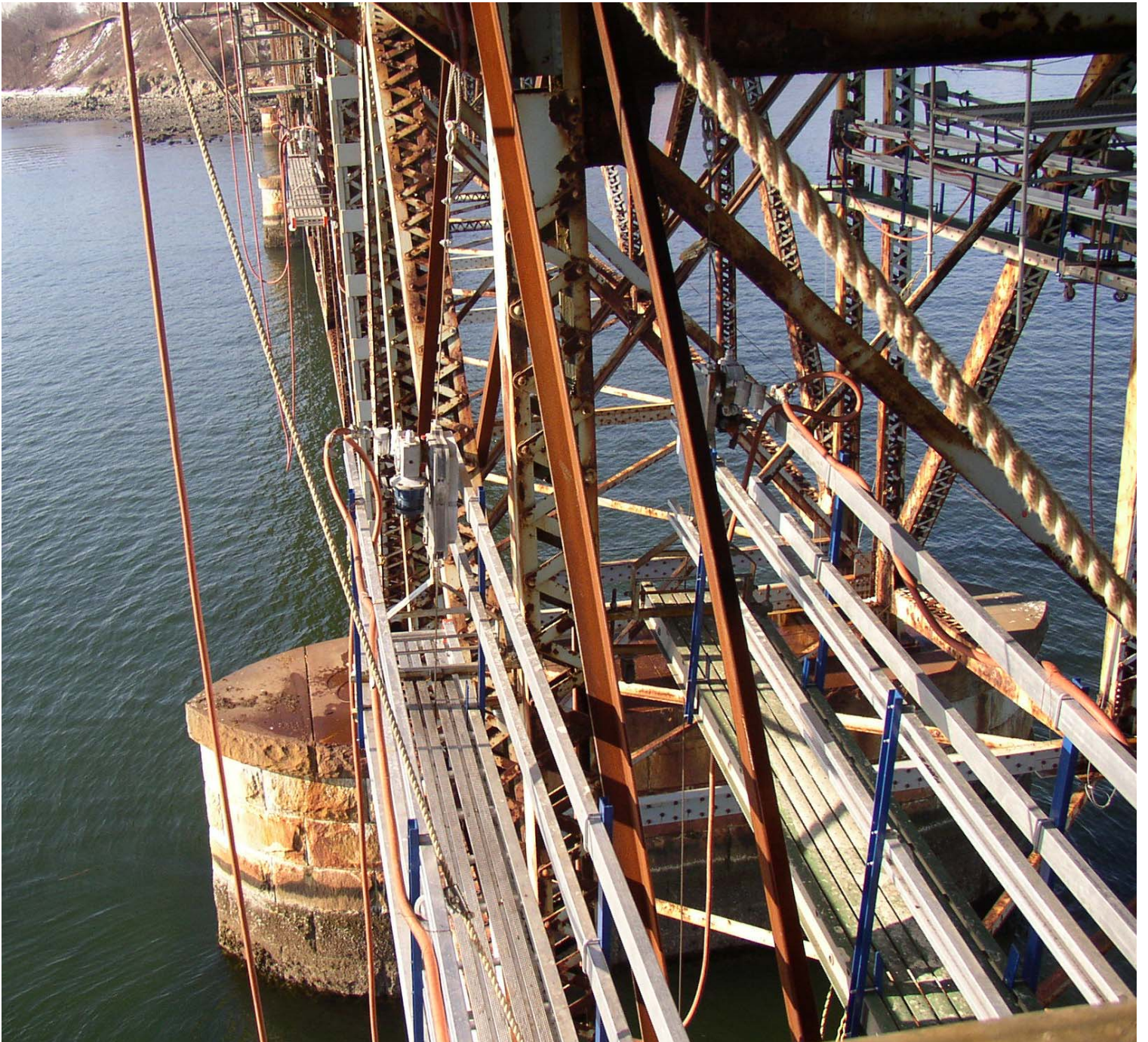
Swing Stage Access System wo/Containment
