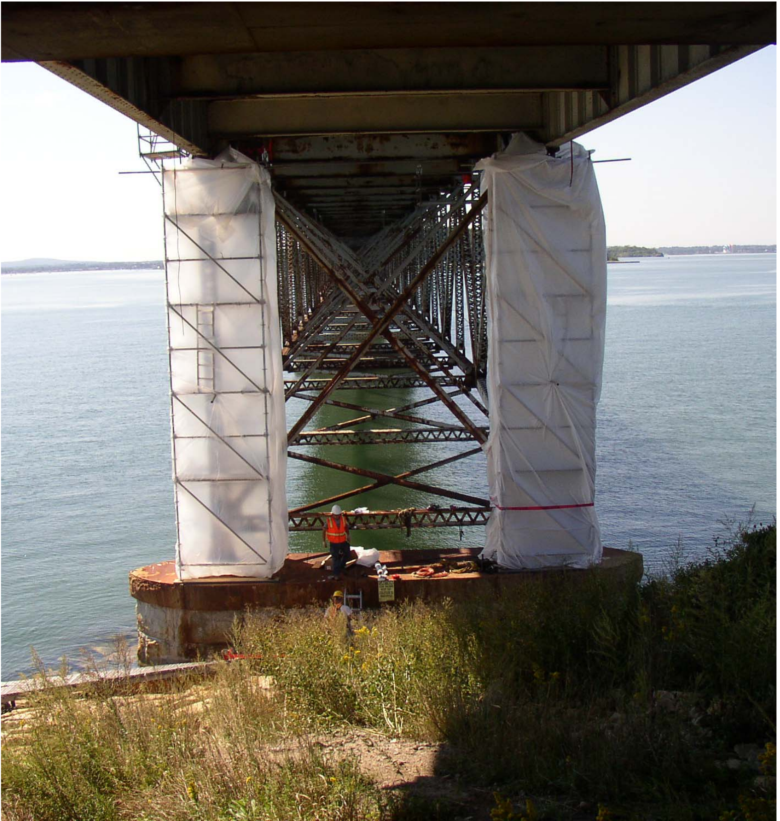
Etobicoke Scaffold Tower System & Containment
