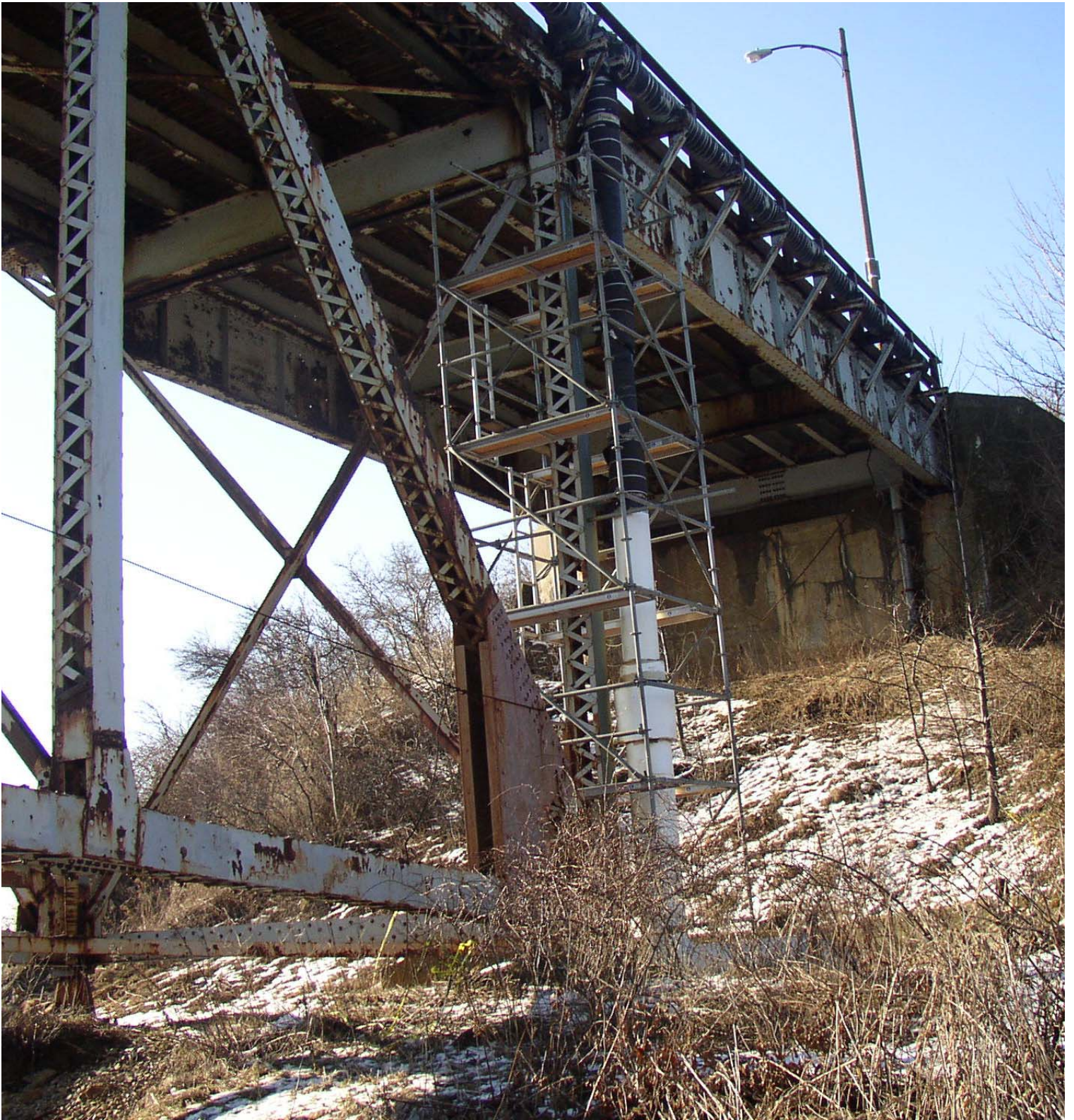
Etobicoke Scaffolding Enclosure
