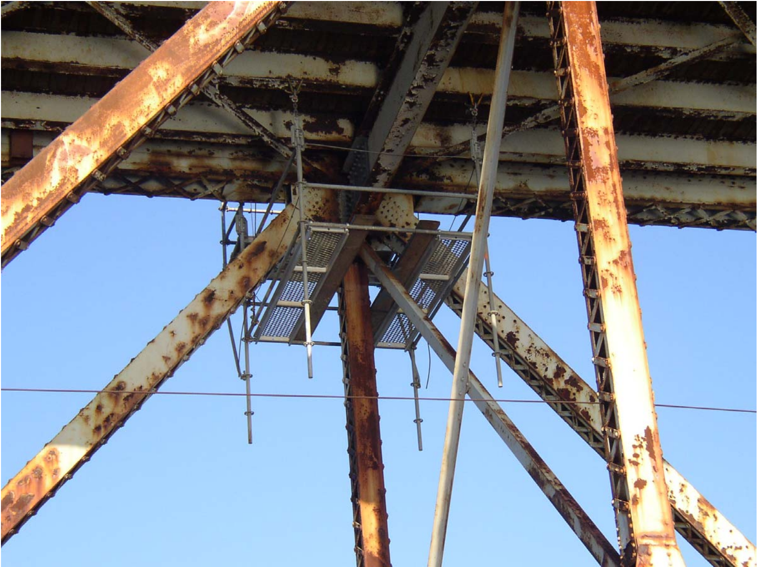
Hanging Etobicoke Scaffold Access System wo/Containment
