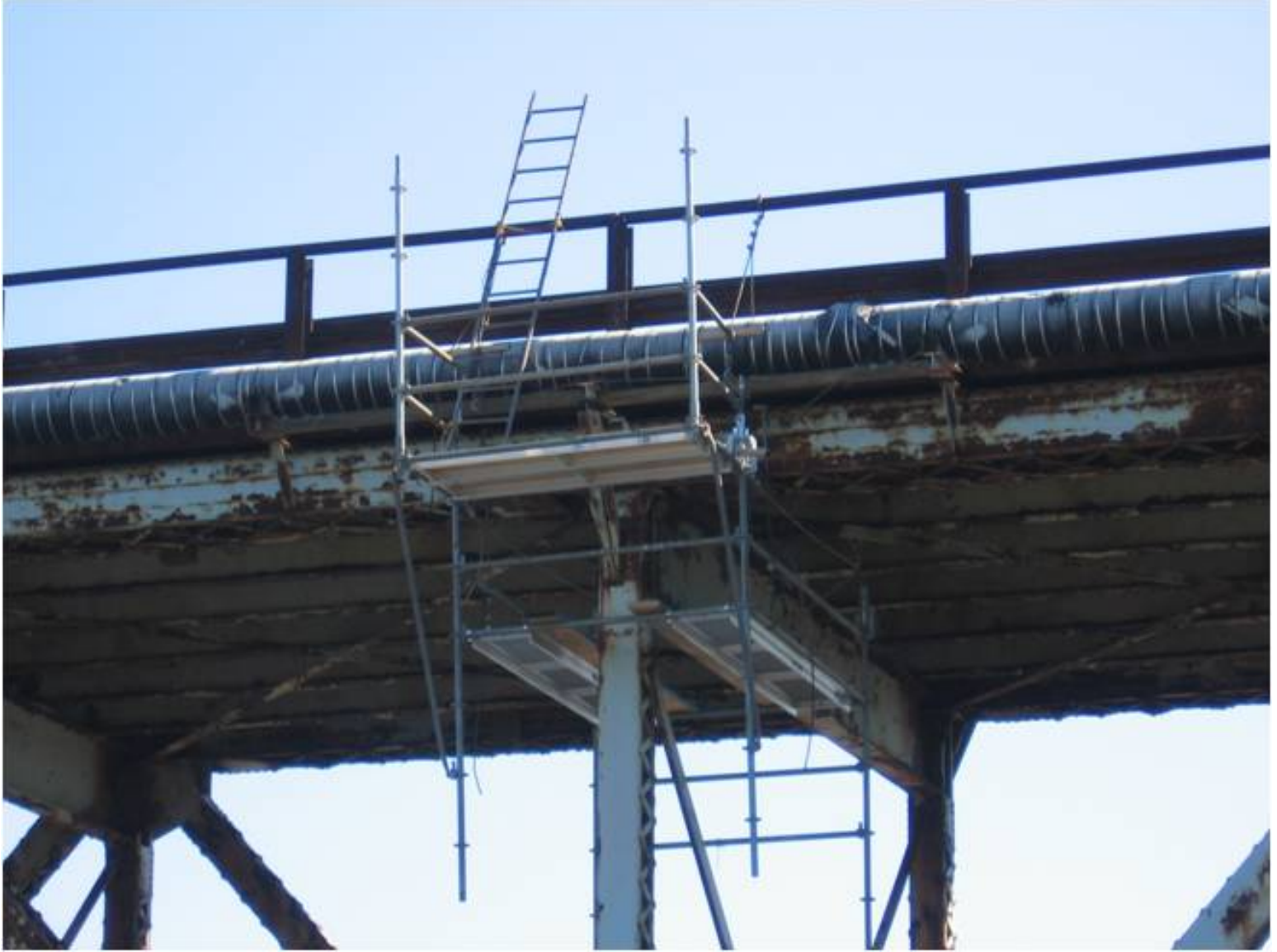
Hanging Etobicoke Scaffold Access System wo/Containment
