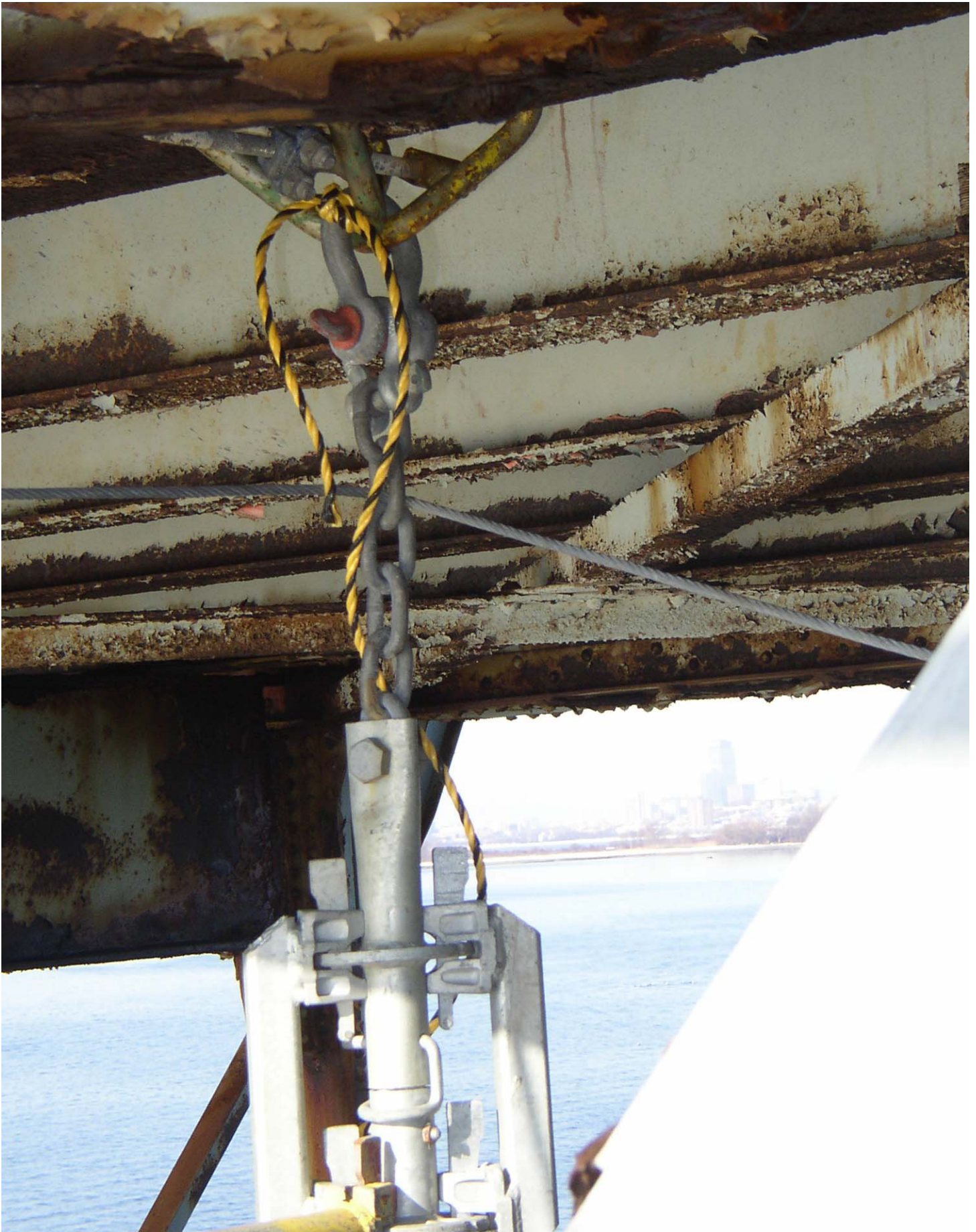
Beam Flange Clamp Hanger Supported Etobicoke Hanger Assembly
