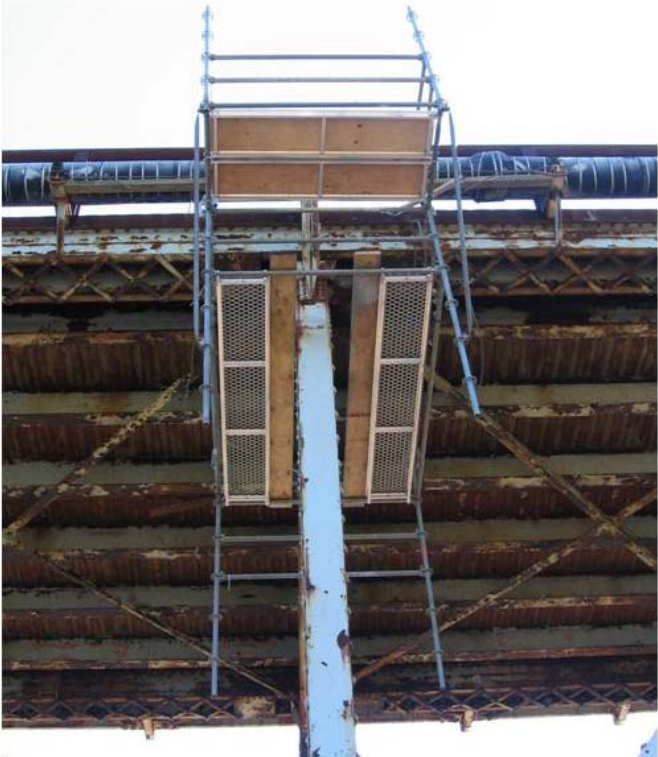
Hanging Etobicoke Scaffold Access System wo/Containment
