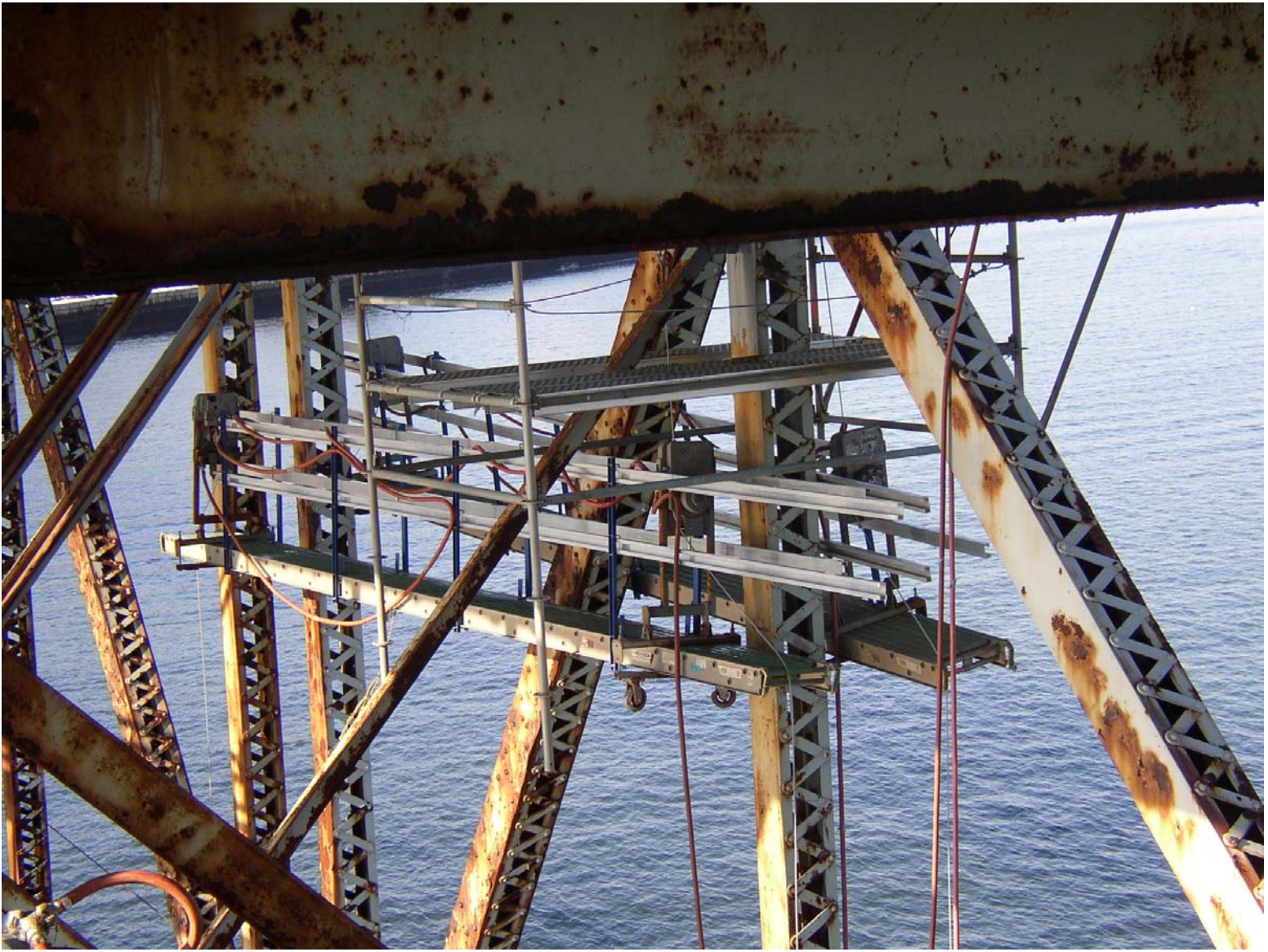
Hanging Etobicoke Scaffold Access System wo/Containment
